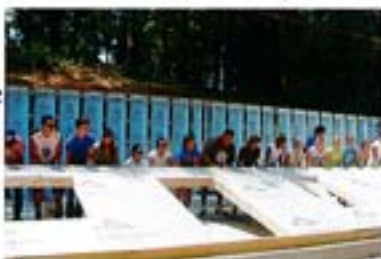
Raising the front wall!
